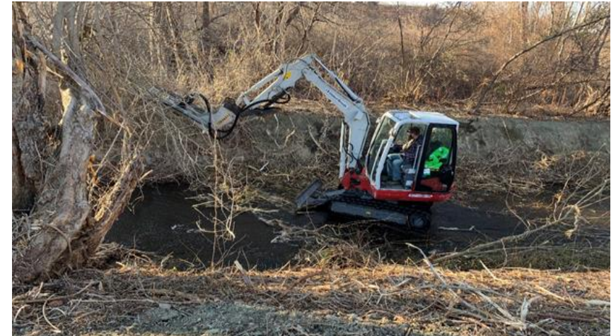
Melville Dam, Portsmouth
