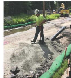
Stateville Public Supply Project - North Smithfield Drinking Water Main Extension.
