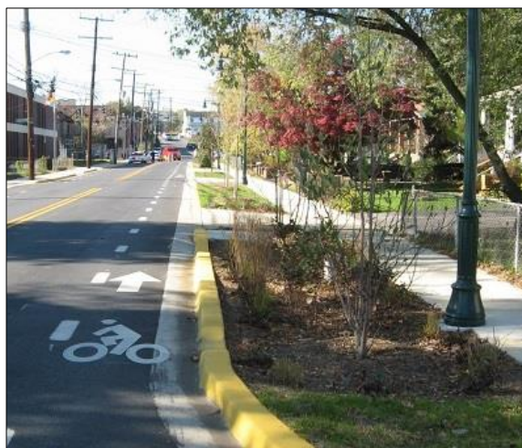
Figure 22: This street in Edmonston, Maryland, incorporates green infrastructure elements, including pervious paving in the bike lane, while making the street pleasant and safe for all users.
