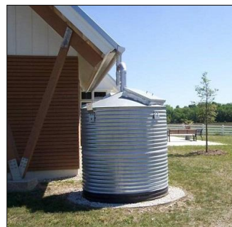
Figure 27: Cisterns can capture runoff from roofs and store it to be used for irrigation or other nonpotable uses
