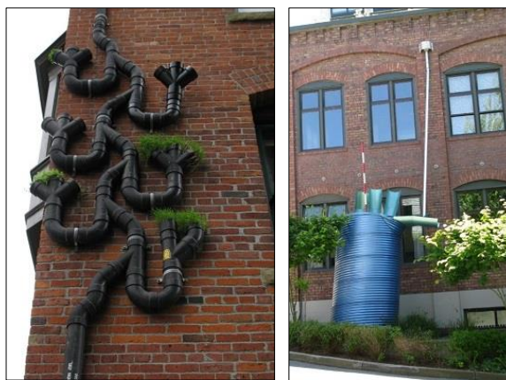
Figure 21: Stormwater-capture devices, such as these in Seattle, can be artistic as well as functional.
