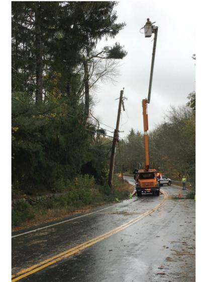
Utility workers repairing damaged power lines in West Kingston
