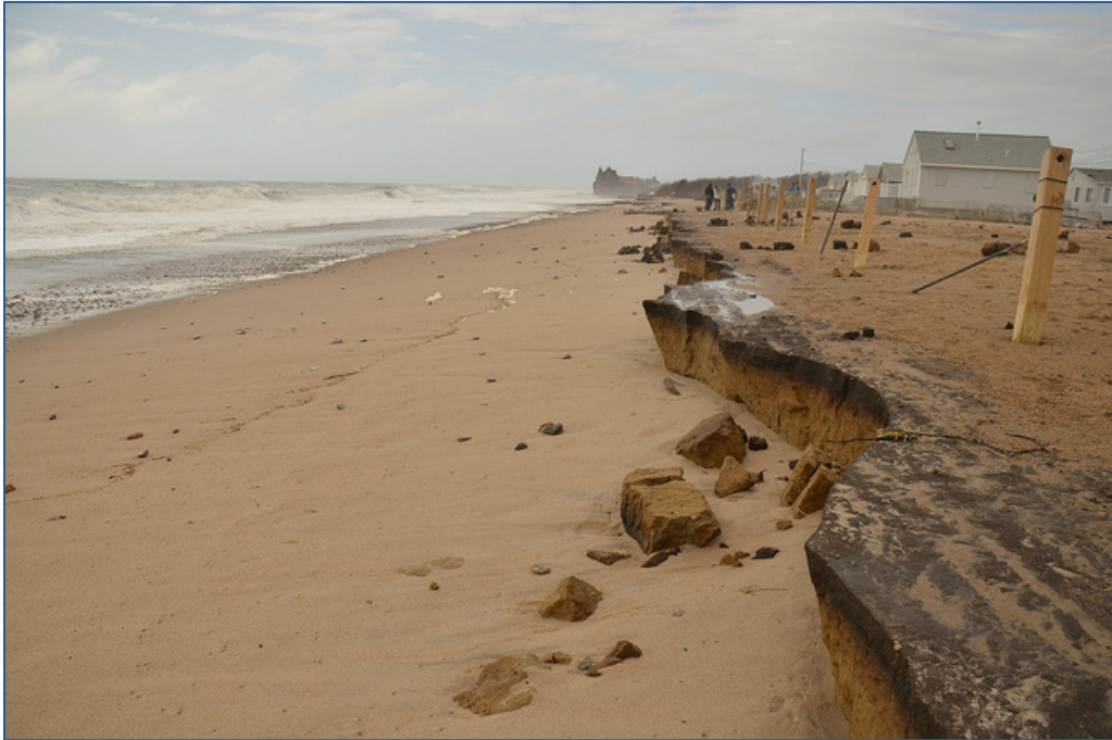
Extensive erosion in Matunuck, R.I. Tropical Storm Sandy caused severe erosion along the southern Rhode Island coast in 2012.
