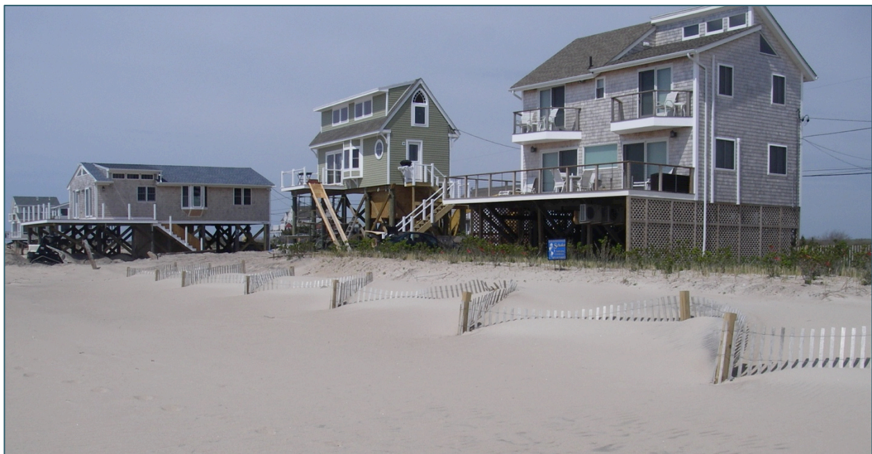
Elevated homes in Westerly, R.I. The green house (center) has been elevated to 5 feet above the base flood elevation.
